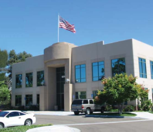
Central San Diego Office
